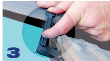
3 SWIVEL CLIP INTO POSITION OVER TILE & PRESS CLIP FIRMLY DOWN INTO WATER COURSE OF TILE
