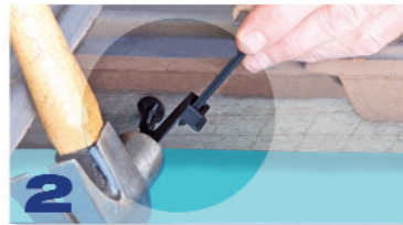
2 HAMMER NAIL INTO BATTEN
