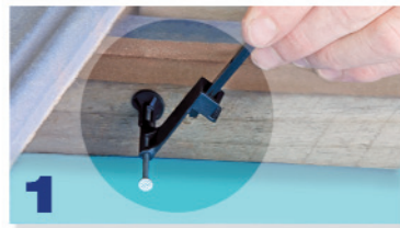
1 POSITION CLIP AT 10° ANGLE AWAY FROM TILE EDGE
